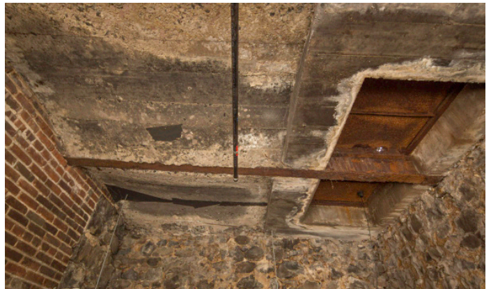
4324 - Ceiling, North Side
