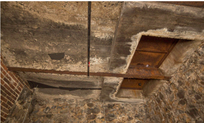
4323 - Ceiling, North Side
