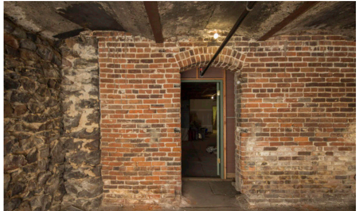
4322 - Looking West, South Side
