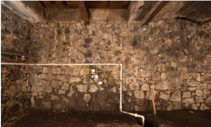
4312 - Looking East, North Side
