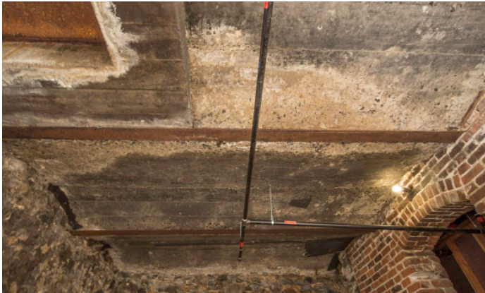
4325 - Ceiling, South Side
