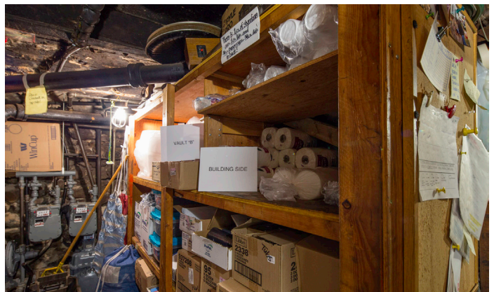
4376 - Building Side Wall
