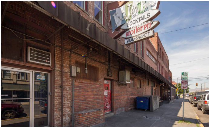
4427 - Outside Sidewalk View
