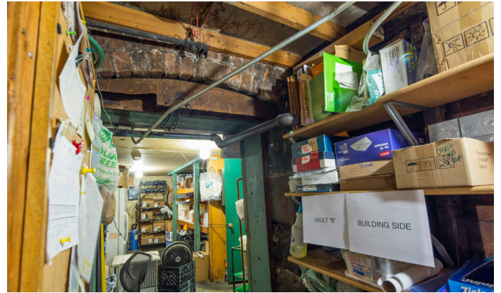
4378 - Building Side Wall
