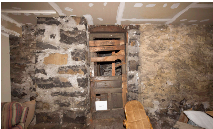
5105 - Vault Door Entry
