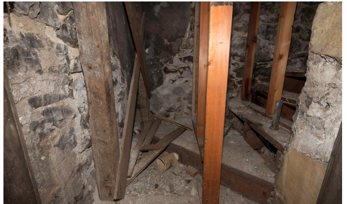
5112 - Door Vault Entry
