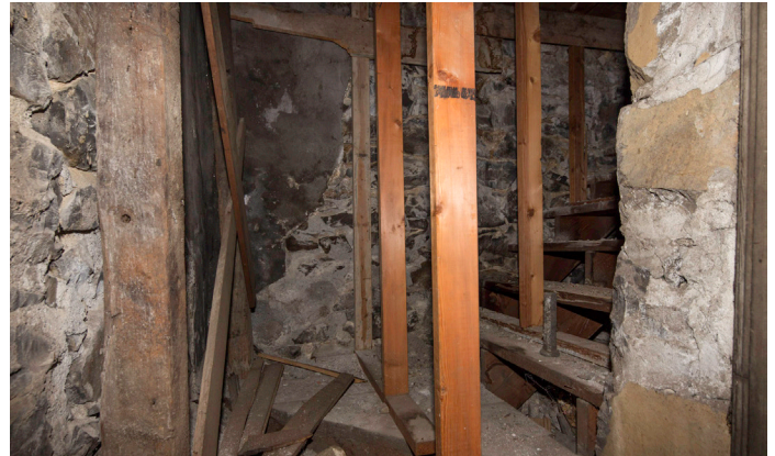
5101 - Street Side, Right Side Wall (Stairs)
