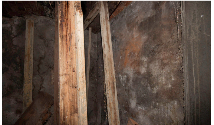
5107 - Right Side Wall
