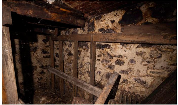
4547 - Right Side Wall
