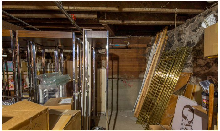
4558 - Looking North to Closed Hatch Door
