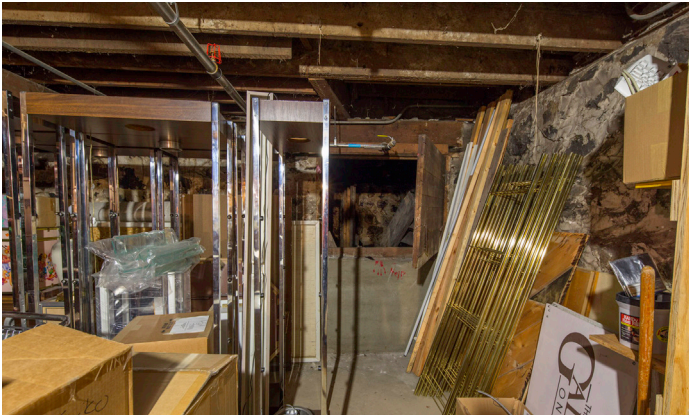
4557 - Looking North to Open Hatch Door
