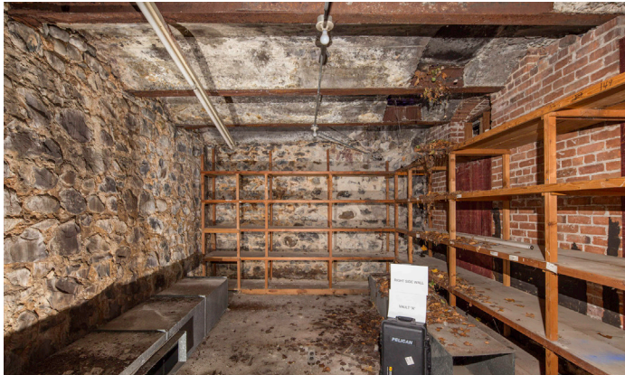
4683 - Right Side Wall
