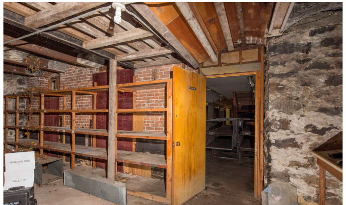
4688 - Building Side Wall
