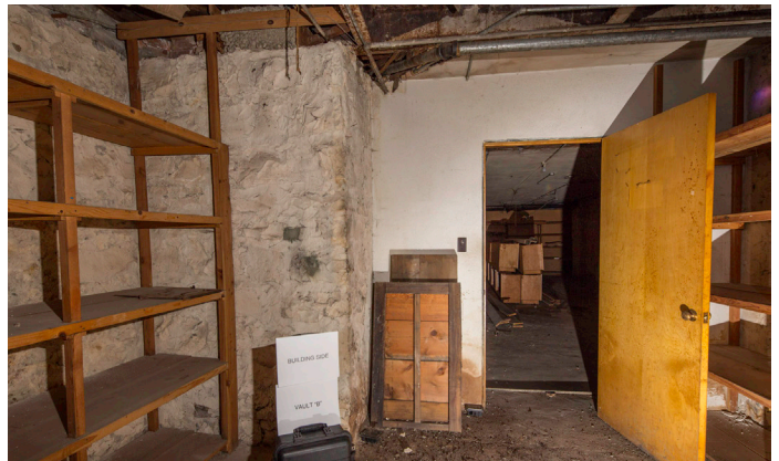
4717 - Building Side Wall
