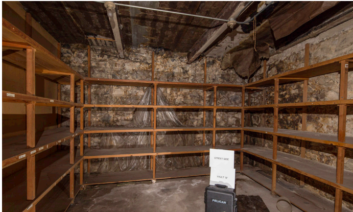
4692 - Street Side Wall
