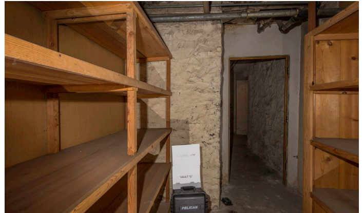
4728 - Building Side Wall
