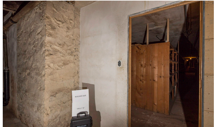
4733 - Building Side Wall
