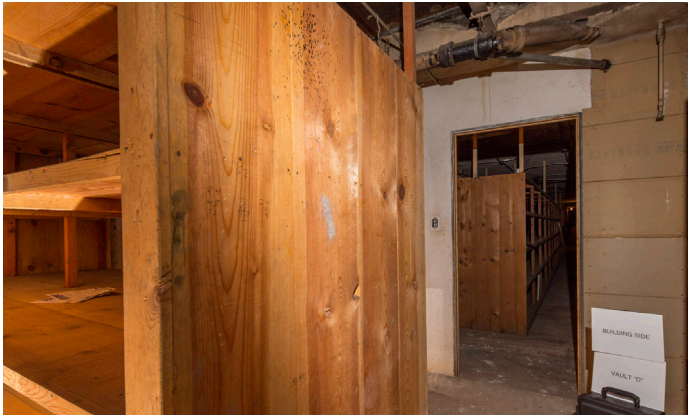
4732 - Building Side Wall
