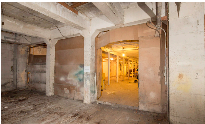
4608 - Vault B, Building Side Wall
