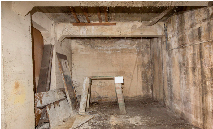
4603 - Vault B, Left Side Wall
