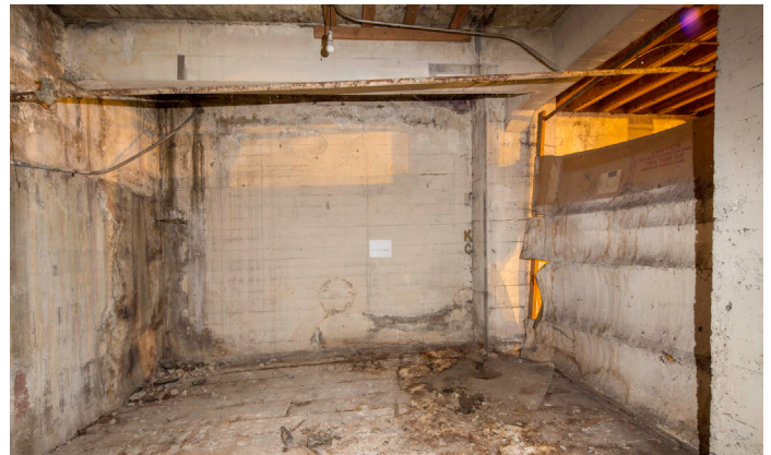
4604 - Vault B, Right Side Wall
