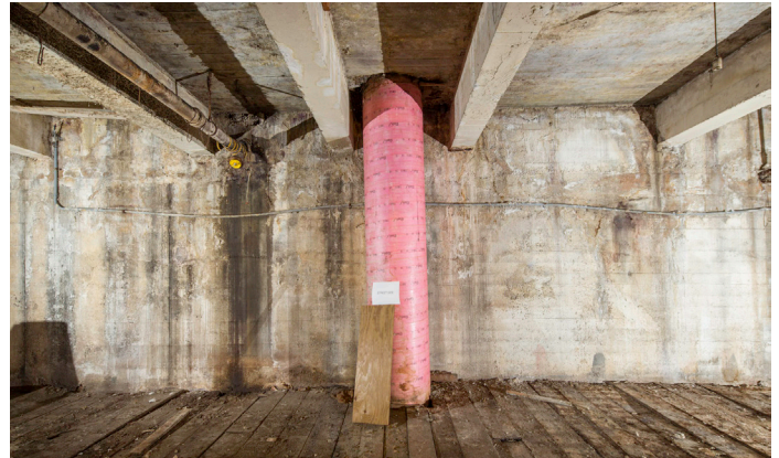
4600 - Vault B, Main Street Side Wall
