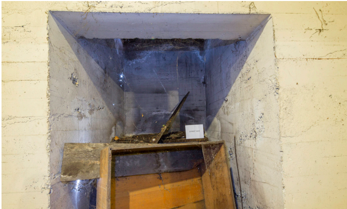
4591 - Vault A, New 6th Street Side Wall
