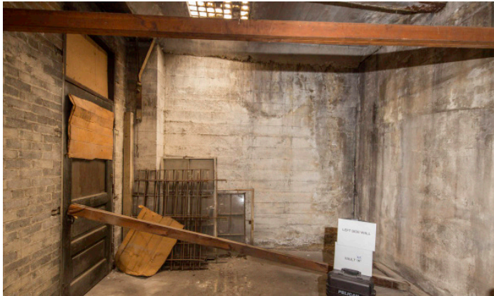
4530 - VAULT AA: Left Side Wall (New 6th)
