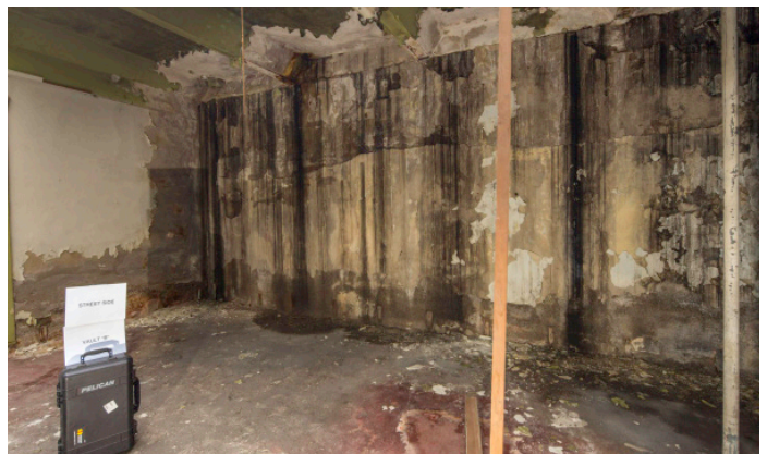
4471 - VAULT B: Street Side (830 Main)
