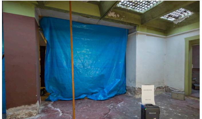
4478 - VAULT B: Building Side (830 Main)
