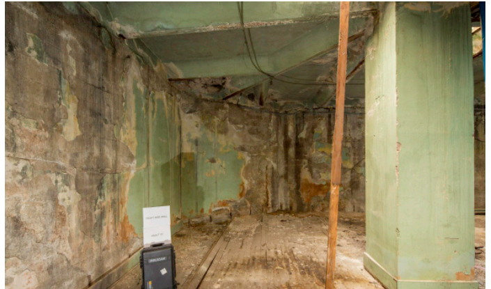
4499 - VAULT C: Right Side Wall (New 6th)
