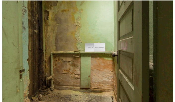
4489 - VAULT B: Right Side Wall (826 Main)
