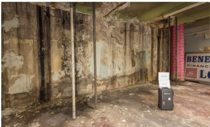
4469 - VAULT B: Street Side (830 Main)
