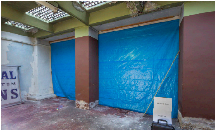
4479 - VAULT B: Building Side (830 Main)
