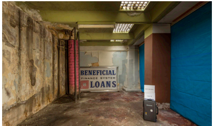
4468 - VAULT B: Right Side Wall (830 Main)
