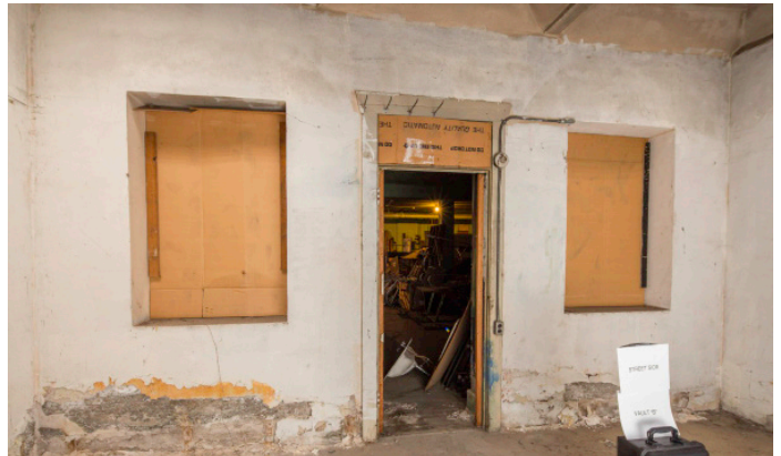
4514 - VAULT B: Street Side (New 6th)
