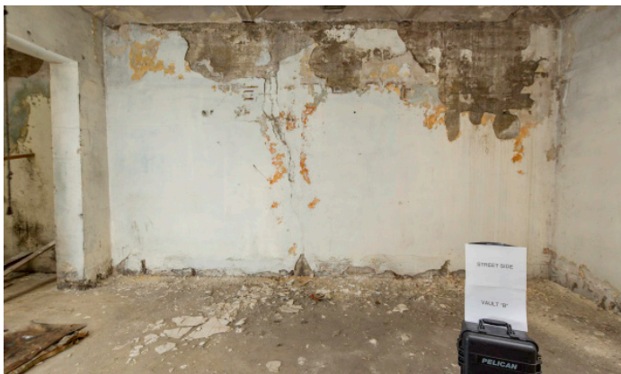
4507 - VAULT B: Street Side (New 6th)
