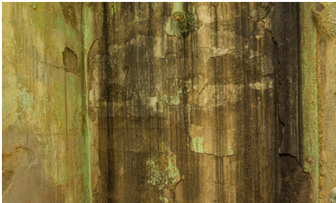
4493 - VAULT B: Street Side (826 Main)
