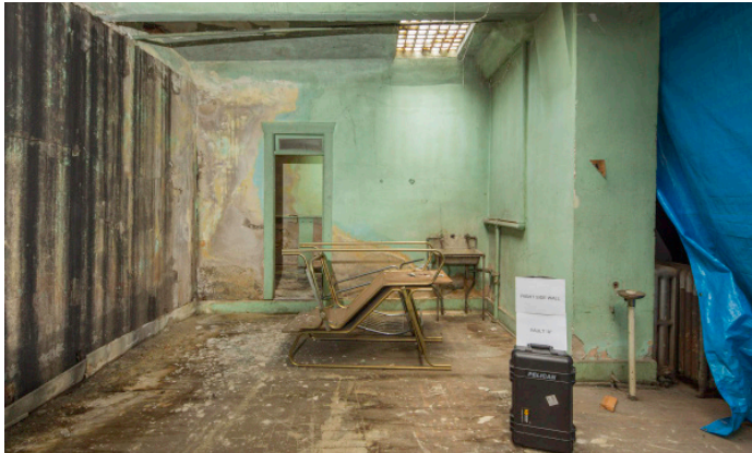
4487 - VAULT A: Right Side Wall (826 Main)
