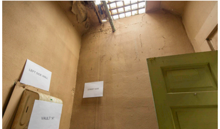
4463 - VAULT A: Left Side Wall, Street Side (830 Main)
