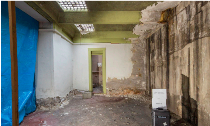
4476 - VAULT B: Left Side Wall (830 Main)
