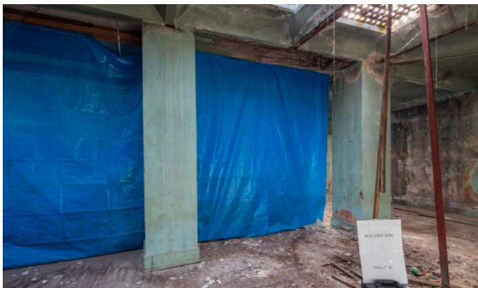
4481 - VAULT A: Building Side (826 Main)
