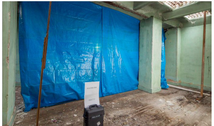
4504 - VAULT C: Building Side (New 6th)
