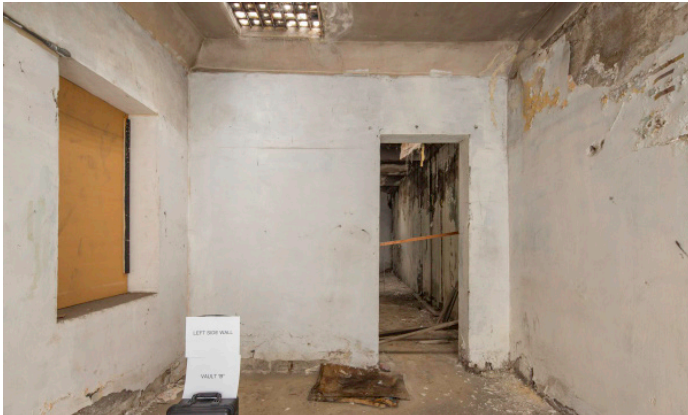
4513 - VAULT B: Left Side Wall (New 6th)
