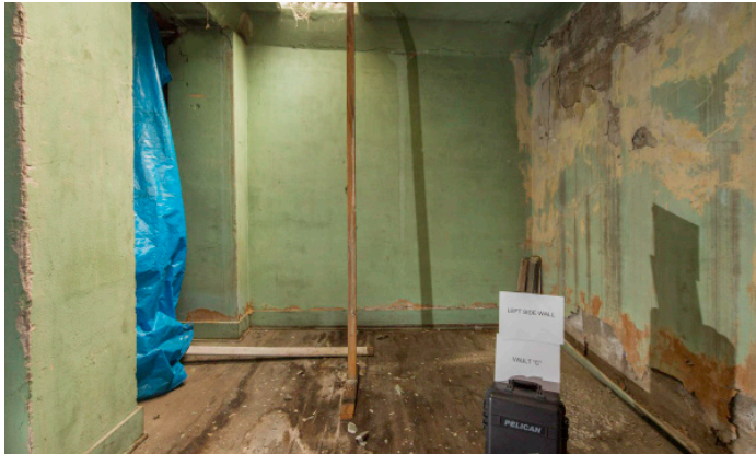
4498 - VAULT C: Left Side Wall (New 6th)
