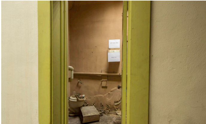
4462 - VAULT A: Left Side Wall (830 Main)
