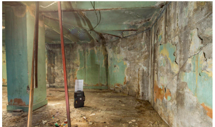
4480 - VAULT A: Left Side Wall (826 Main)
