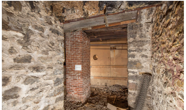
4651 - Building Side Wall
