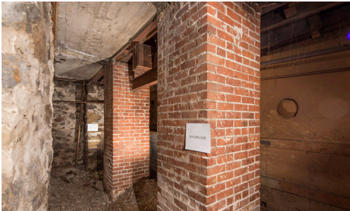
4627 - Building Side Wall
