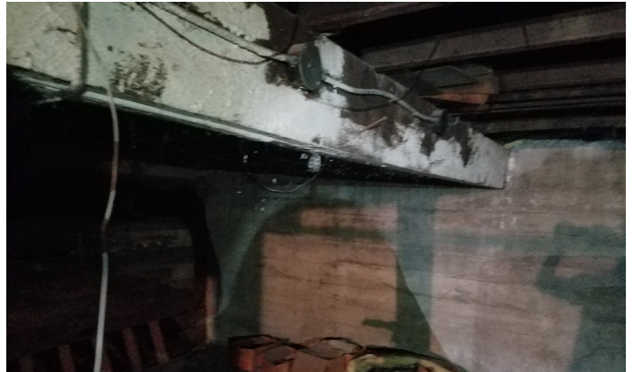
Looking North at Street Side, Left Side
