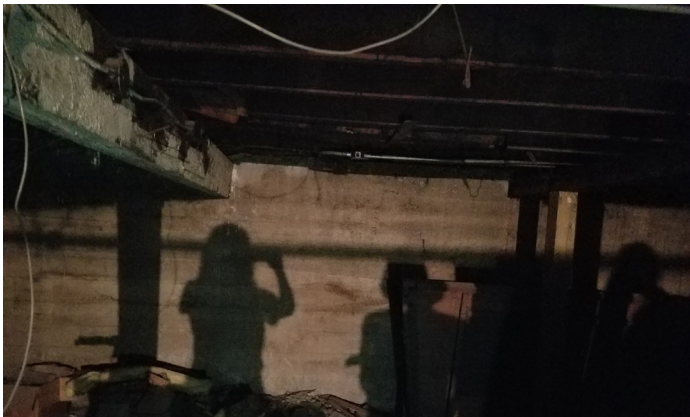
Looking North at Street Side
