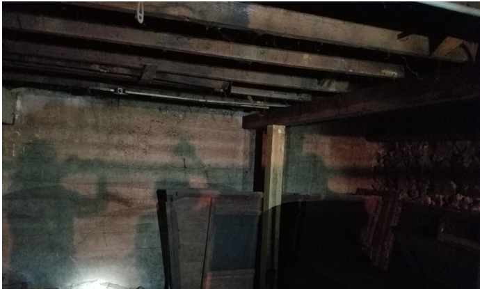
Looking North at Street Side, Right Side
