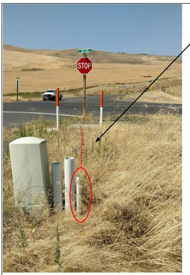
Connect 2" conduit to existing POL HH at the intersection of Wall St. and SH 128.
