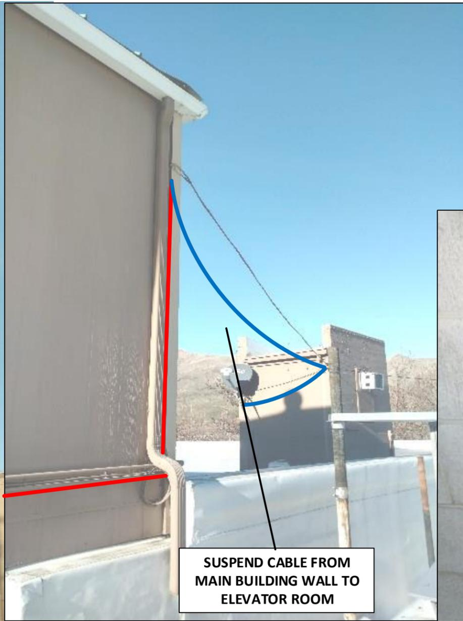
SUSPEND CABLE FROM MAIN BUILDING WALL TO ELEVATOR ROOM
