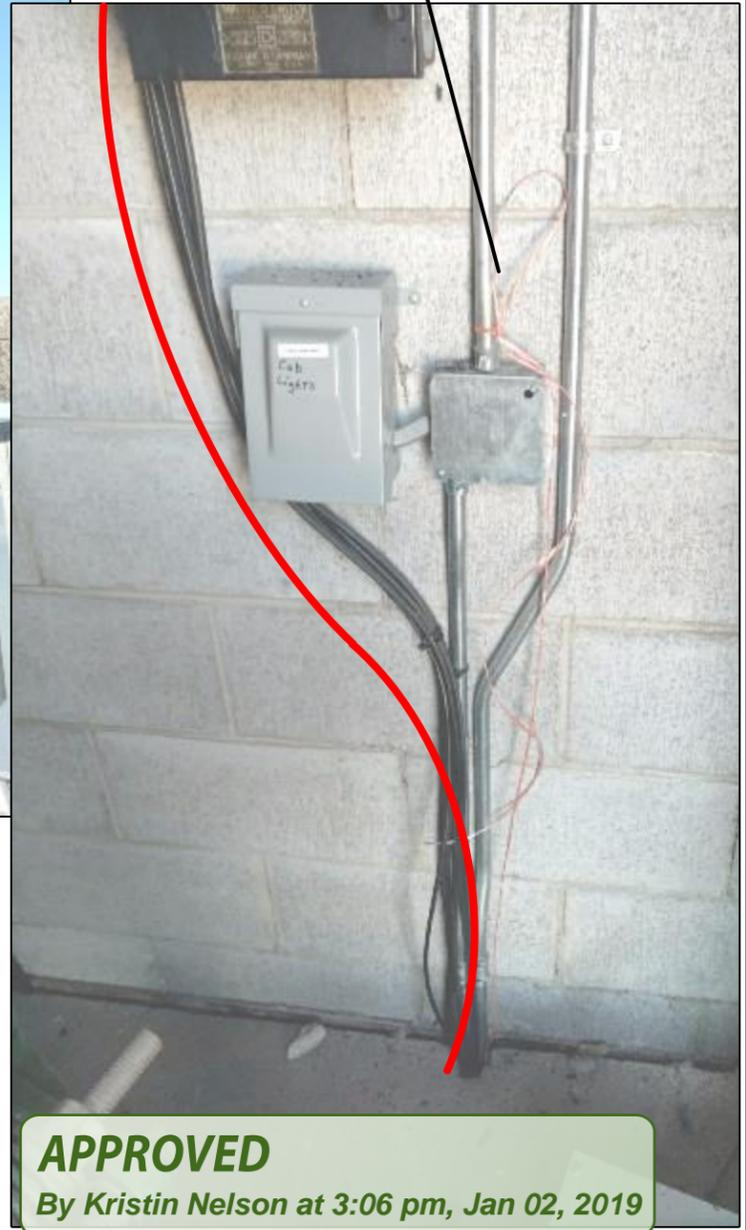
USE EXISTING PULL STRING IN TOP OF ELEVATOR ROOM TO PULL CABLE TO STREET LEVEL FLOOR SERVER ROOM
