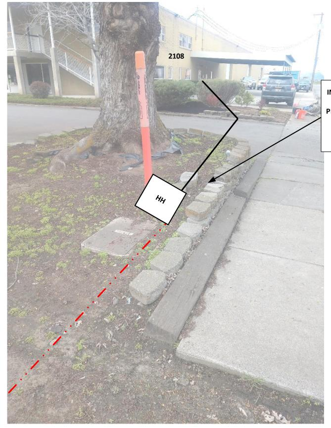
INTERCEPT EXISTING CONDUIT ON WEST SIDE OF CTL HH. PLACE NEW HH OVER EXISTING CONDUIT AND ROD FIBER CABLE THROUGH EXISTING CONDUIT INTO BUILDING.
